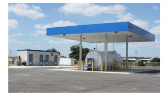
One of the first challenges is deciding between above ground storage tanks (AST) or underground storage tanks (UST), as each style of tank has its pros and cons.
